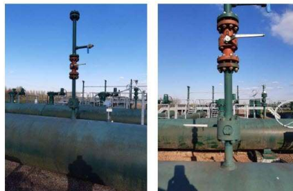
Figure 4. Details of tapping point used in trial
